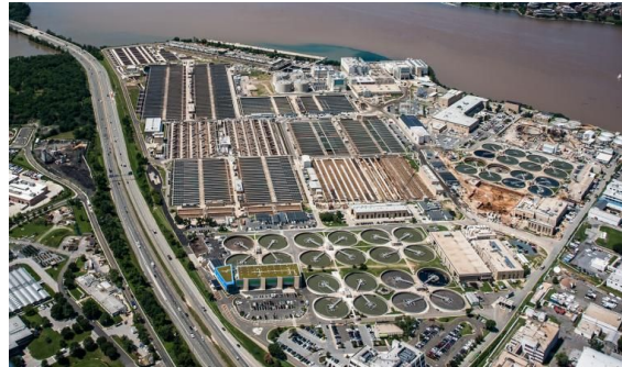
Blue Plains Advanced Wastewater Treatment Plant (photo credit: DC Water)
