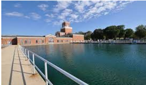
McMillan Water Treatment Plant (photo credit: DC Water)
